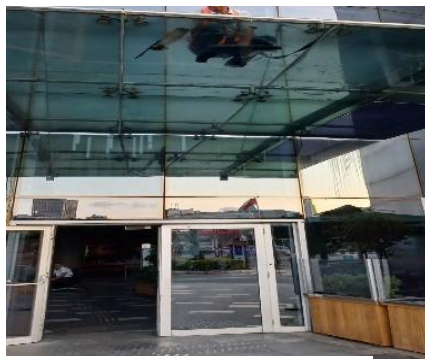
Figure 6. A glass porch without a lifeline Source: Author's own work.
