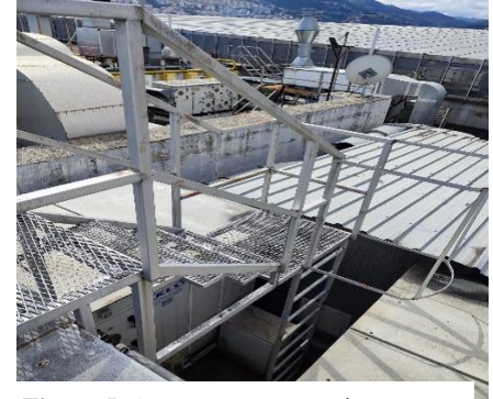
Figure 5. A secure access road on a rooftop area (sample application) Source: Author's own work.
