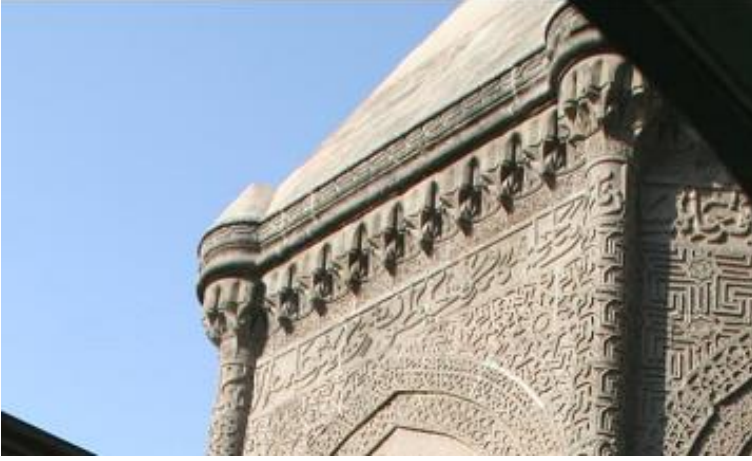
Figure 19. Detail of the Inscriptions and Decorations on the Mausoleum Source: Blessing, 2014
