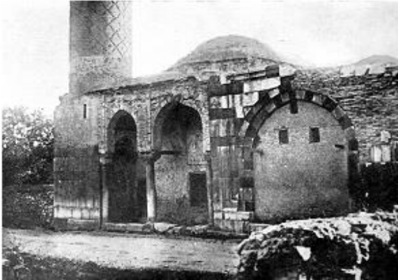
Figure 6. Entrance Facade of Akşehir Taş Madrasa Source: Kuran, 1969
