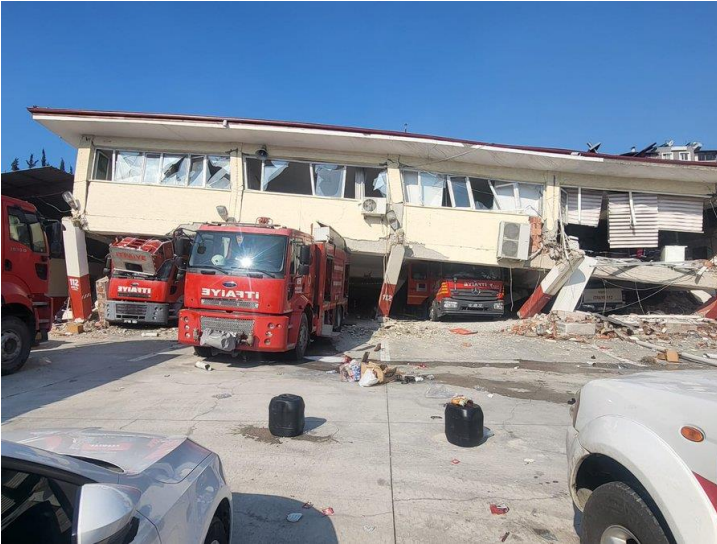
Picture 2: Hatay Fire Brigade damaged in the earthquake
